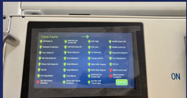
High voltage battery alarm
